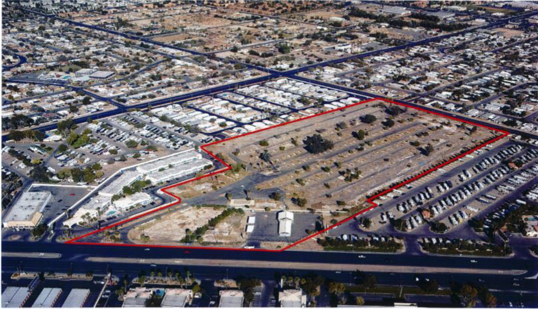
Proposed Site for Boulder Highway Collaborative Campus. Source: Clark County Board of Commissioners
